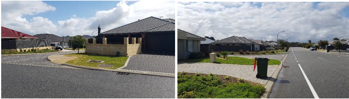
Photos 1 & 1a: Typical corner lot driveways, at the transition point from semi- to mountable kerbs.
