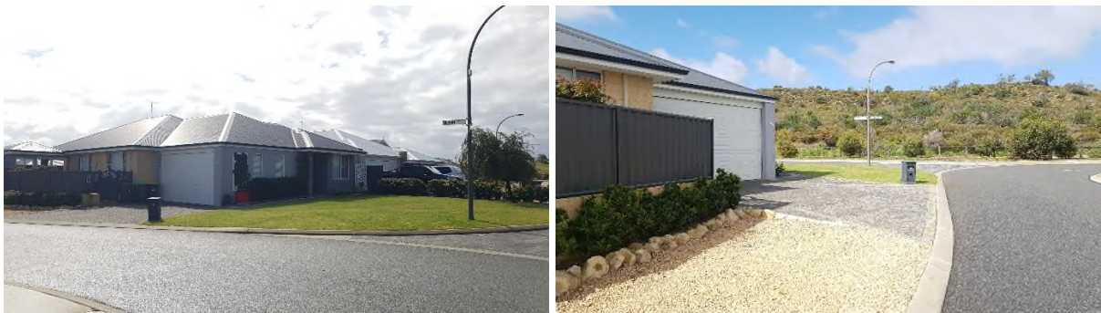
Photos 2 & 2a: Typical corner lot driveways onto primary street, within the mountable kerb section.
